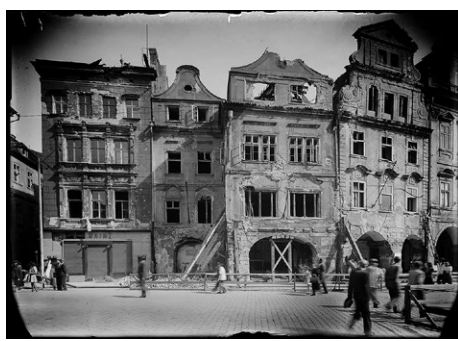
7. Houses on the Southwest Side of Old Town Square Address: Staroměstské náměstí 483/21, 482/22, 481/23, 480/24, Praha 1 GPS: 50.0868750N, 14.4212039E
